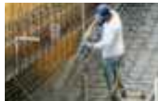
7 to 12 bar: Shotcrete applications
