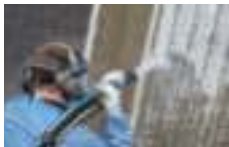
8.6 to 10 bar: Abrasive blasting
